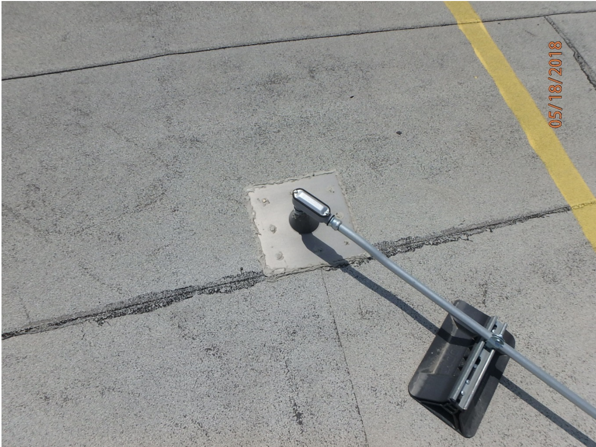
3-course around newly installed pipe flashing per NRCA guide lines
