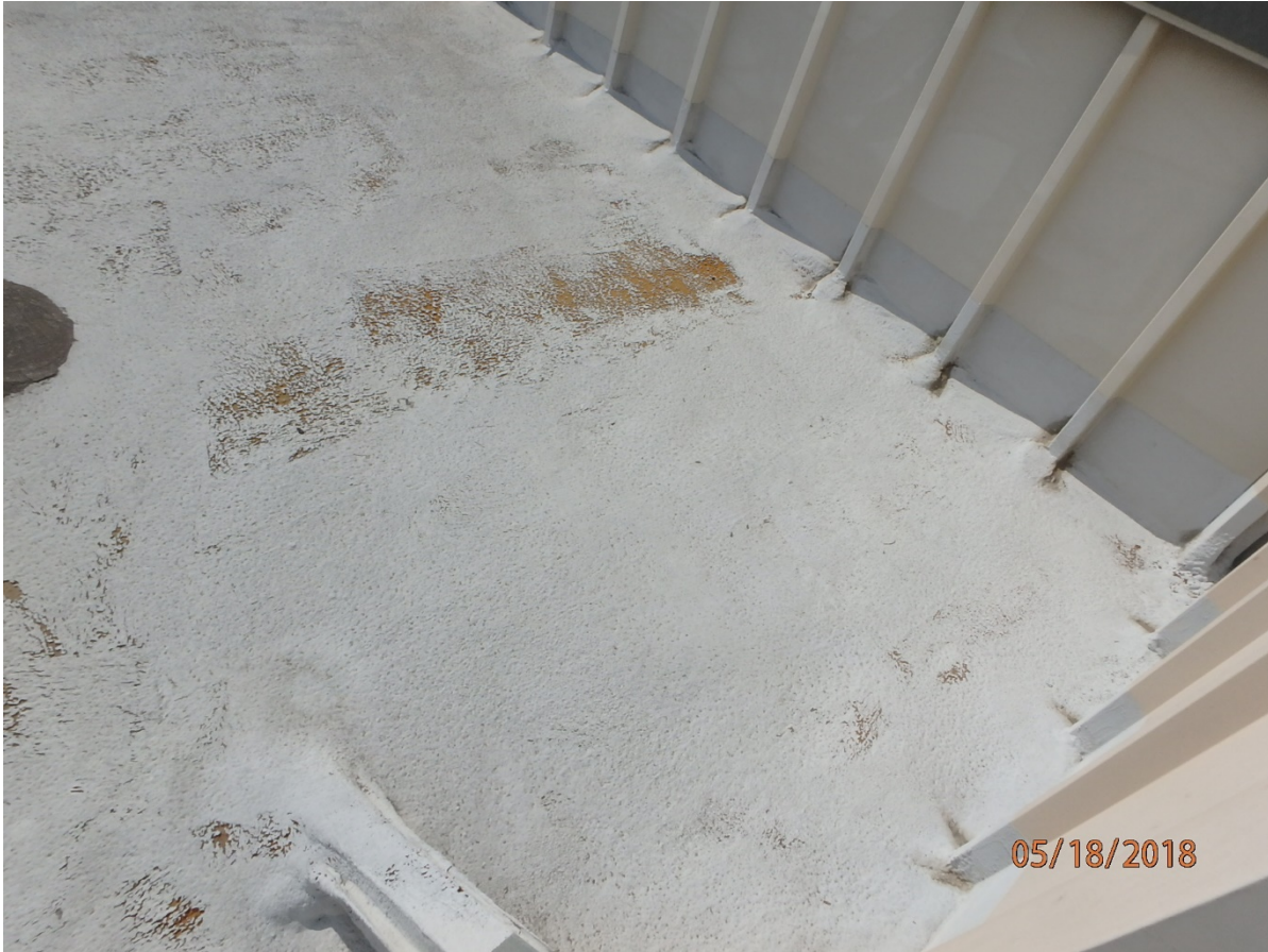
Clean and coat existing SPF roofing
