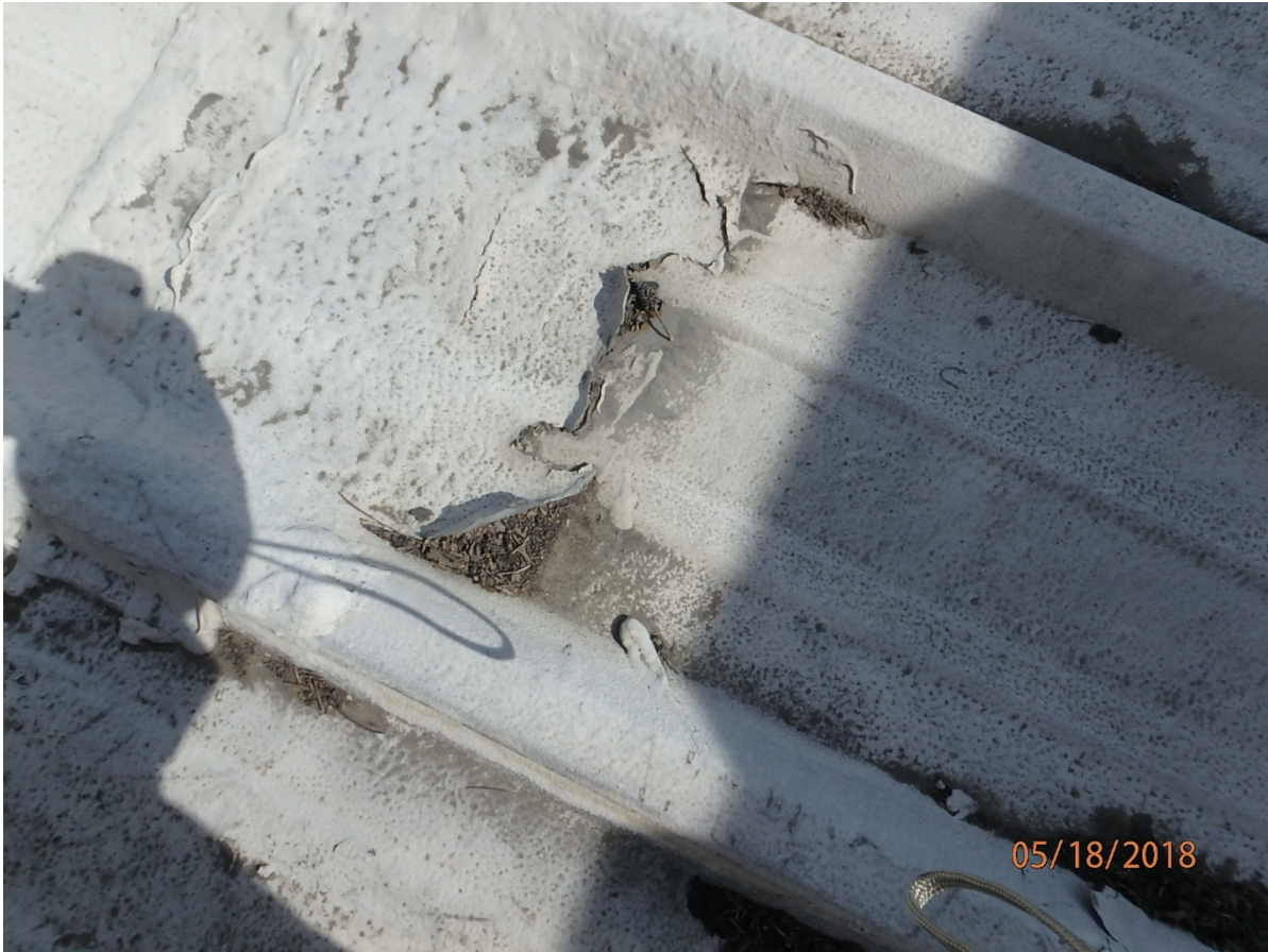
Remove and clean loose coating
