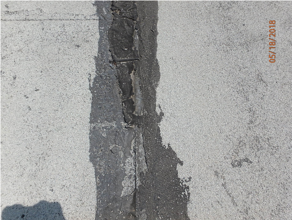
Clean old mastic repairs and apply a 3-course repair
