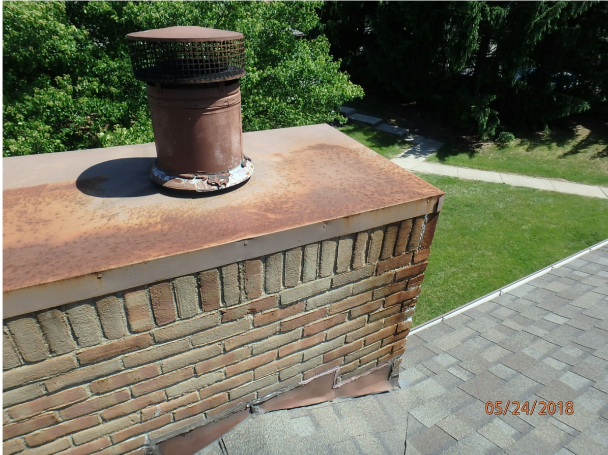
Remove and Replace Chimney chase caps
