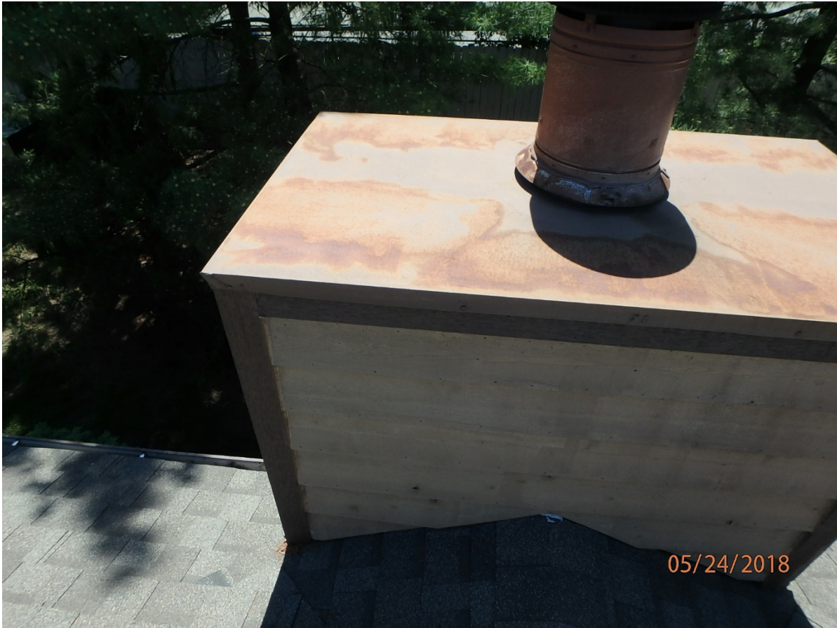
Remove siding to install new step-flashing and raise 1-1/2 to 2 inches above roof
