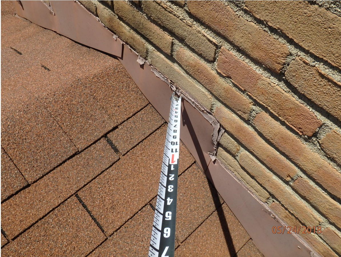
Remove and install new step flashing / Clean ALL old sealant from counterflashing and install new Counter-flashing per NRCA guide lines
