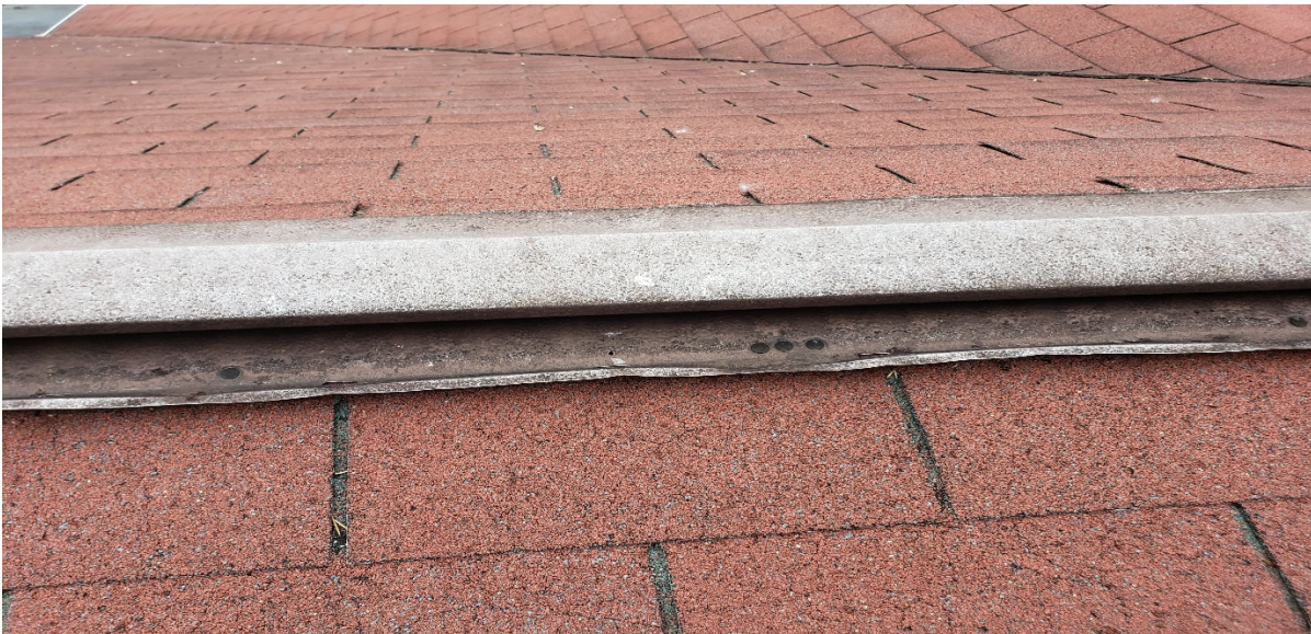
Remove and Replace Static vents and Ridge Vents as needed
