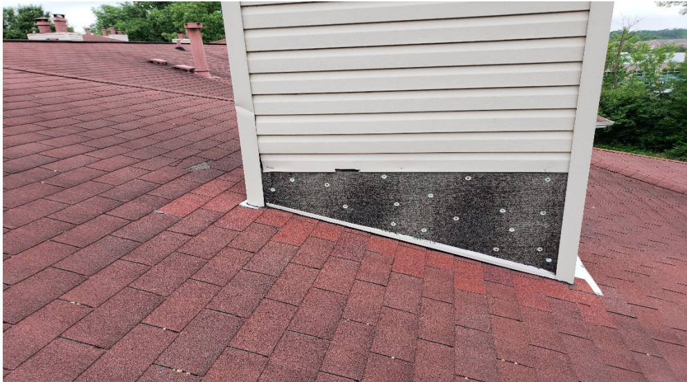
Replaced missing Vinyl siding
