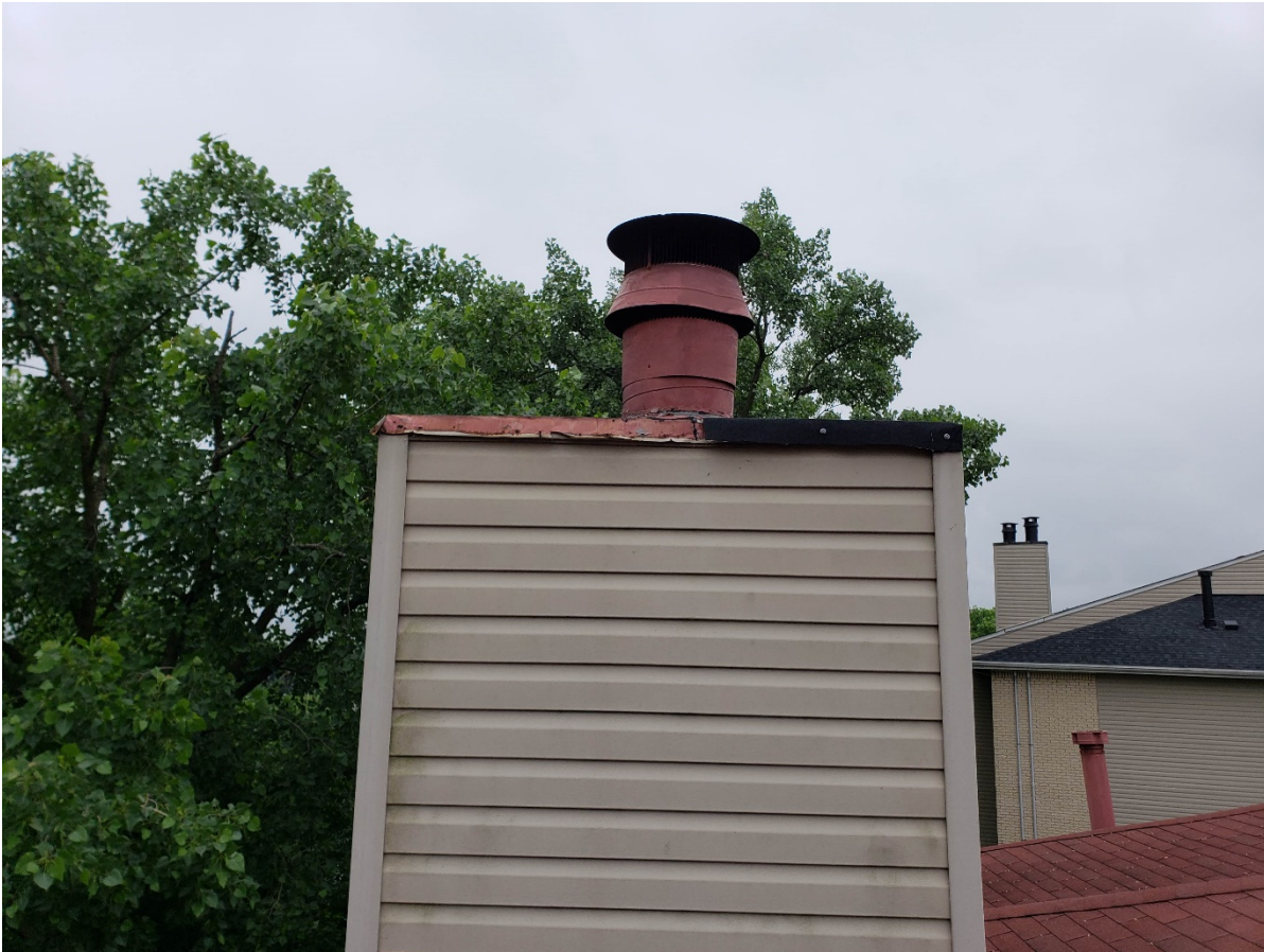
Replace damage Chimney caps
