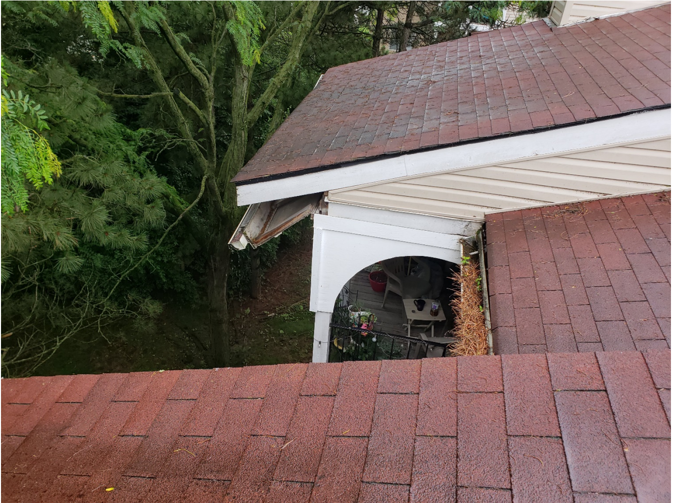
Repair loose and damage soffit
