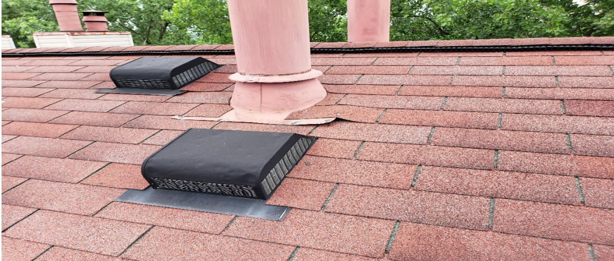
Remove and Replace Static vents and Ridge Vents as needed
