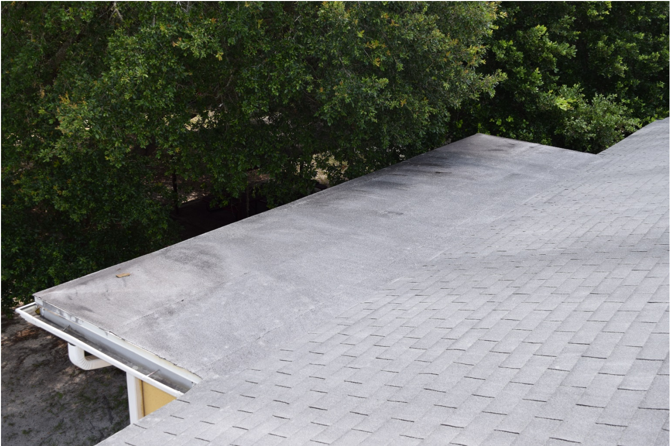
Low slope roof to be included in re-roofing project
