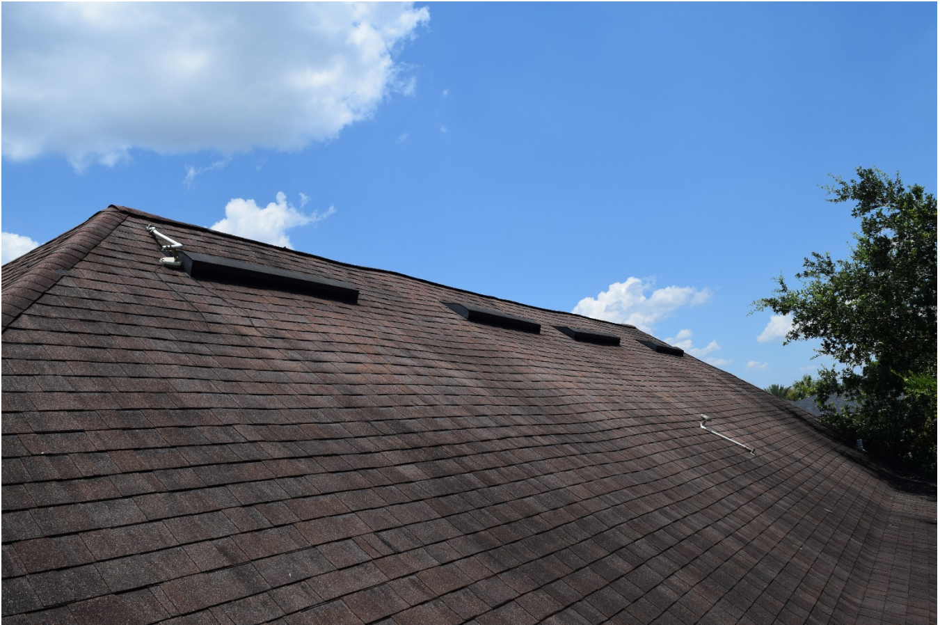
Remove existing dormer vent clean, prime and repaint Reuse existing dormer vents
