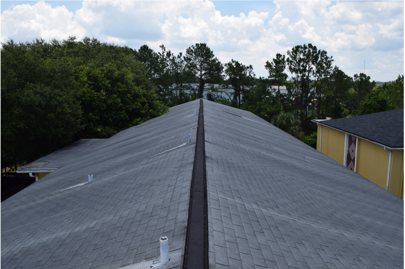
Replace ridge venting
