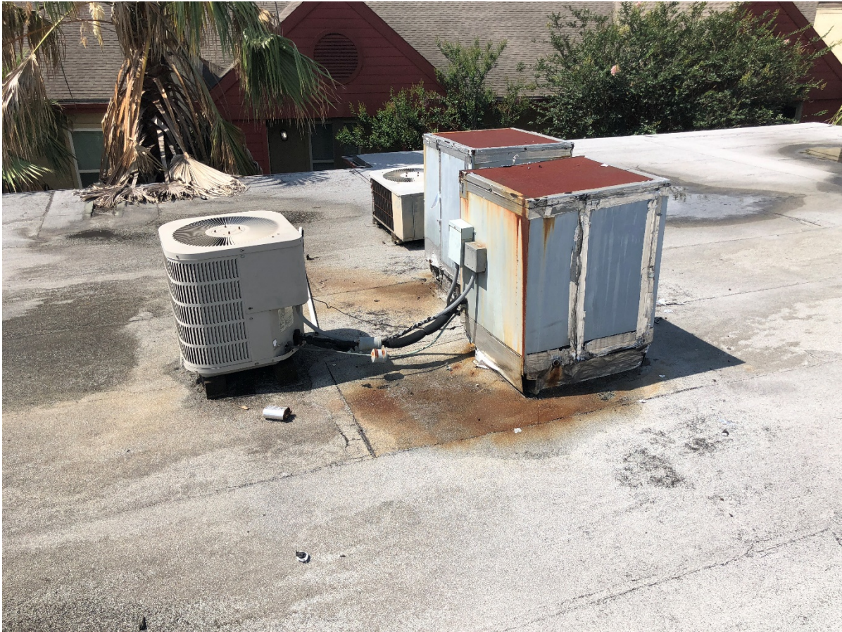
Clean debris off of roofs
