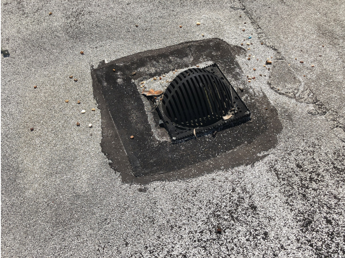
Clean around drains and apply a 3-course patch around lap seams
