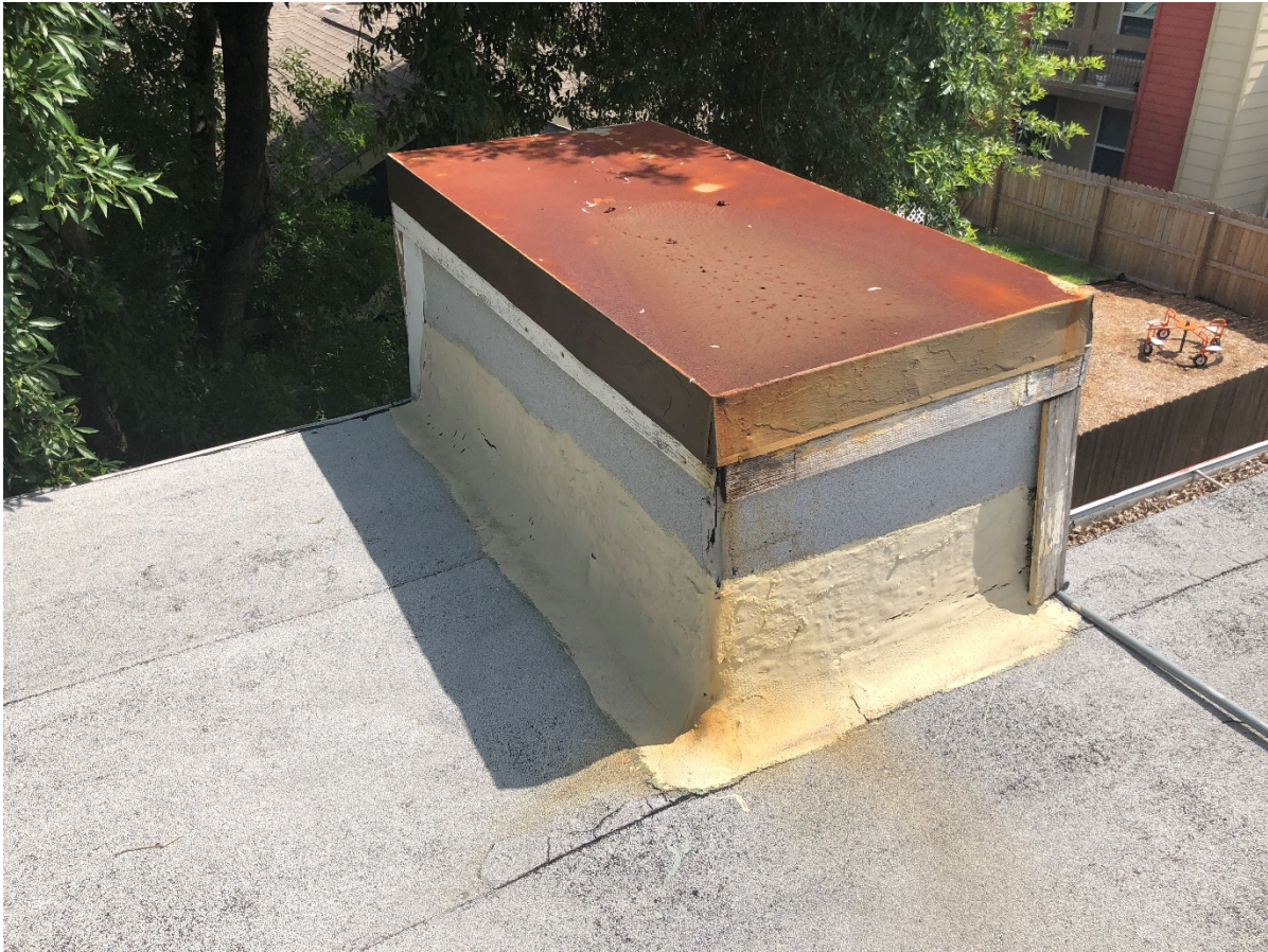
Replace sheet metal caps
