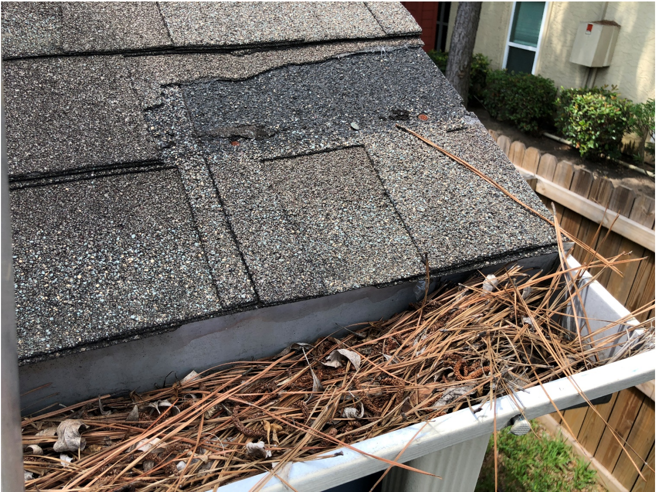
Repair missing or damage shingles to match existing shingles
