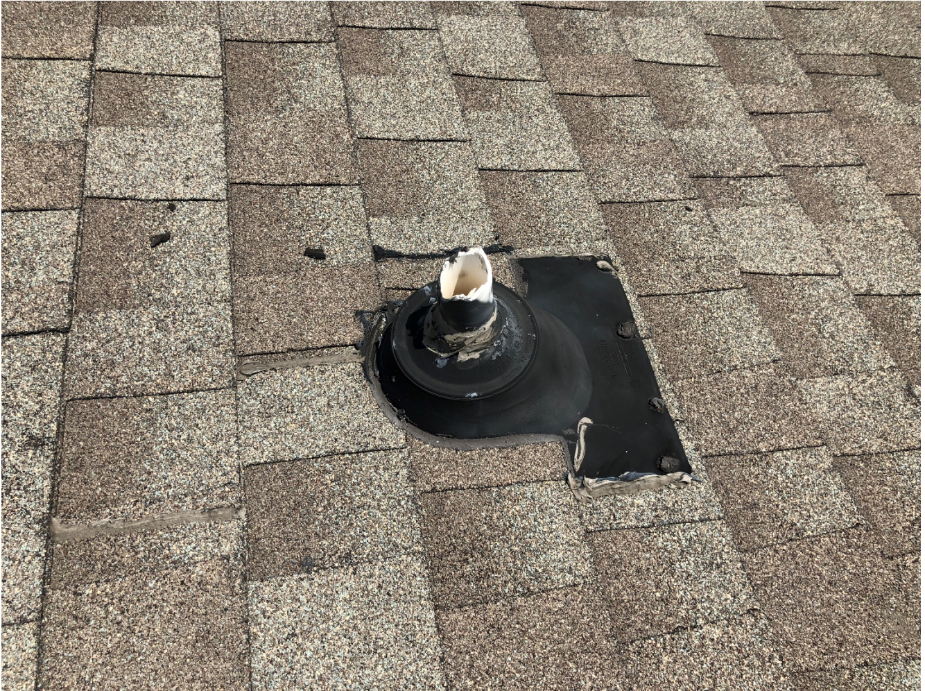
Extend broken vent pipes
