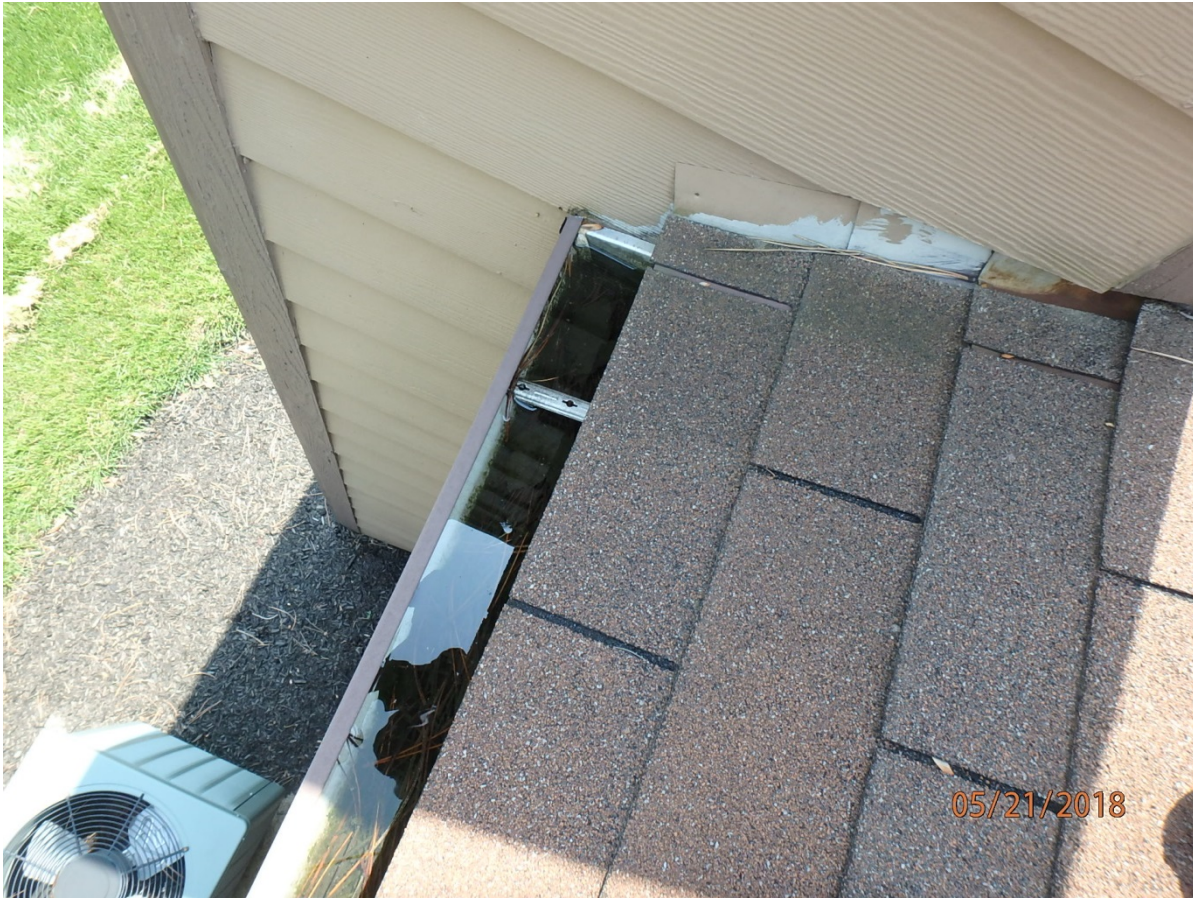
Make sure ALL Step Flashing is counter-flashed
