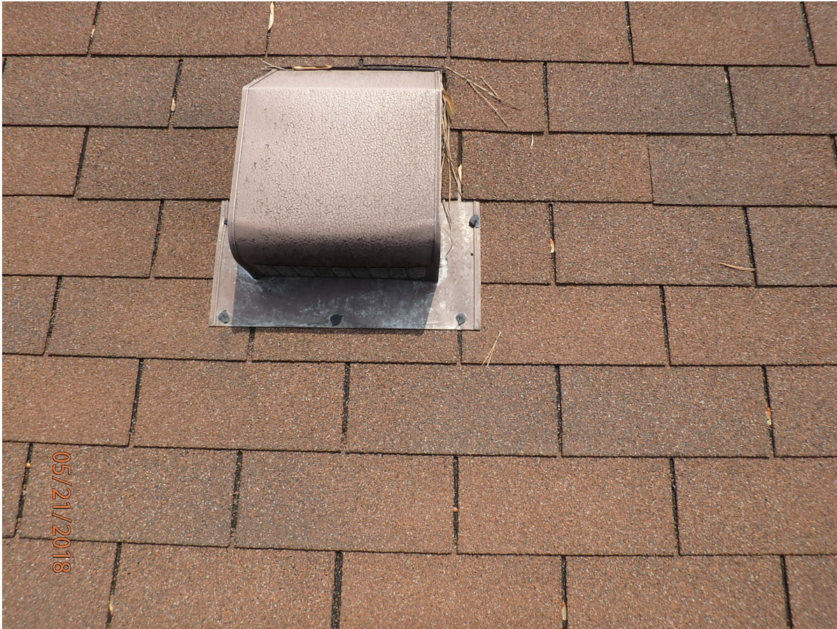
Reuse static vents / Clean, prime and paint to match Shingles
