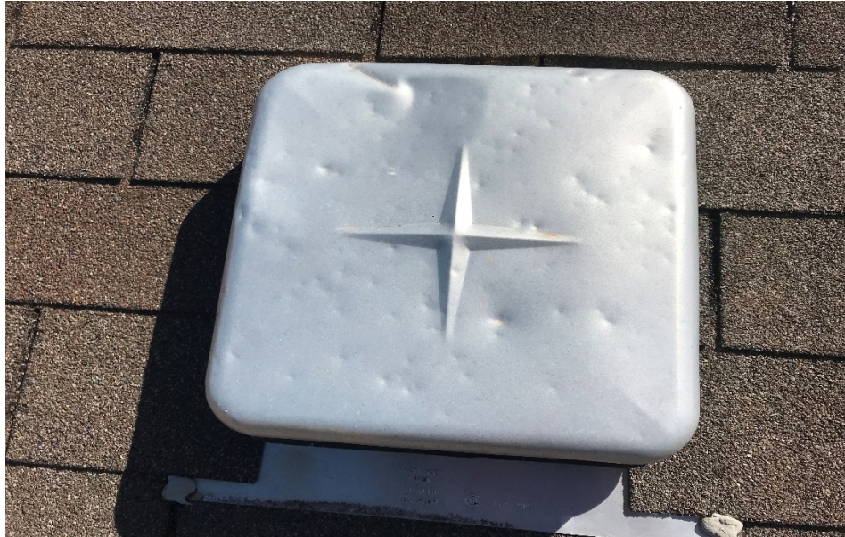
Remove and Replace Static vents and Ridge Vents as needed
