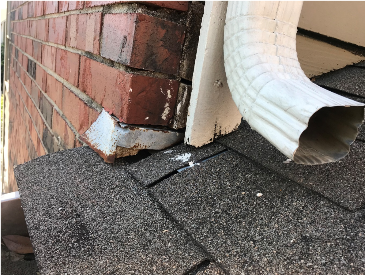
Install new metal flashing and set with sealant
