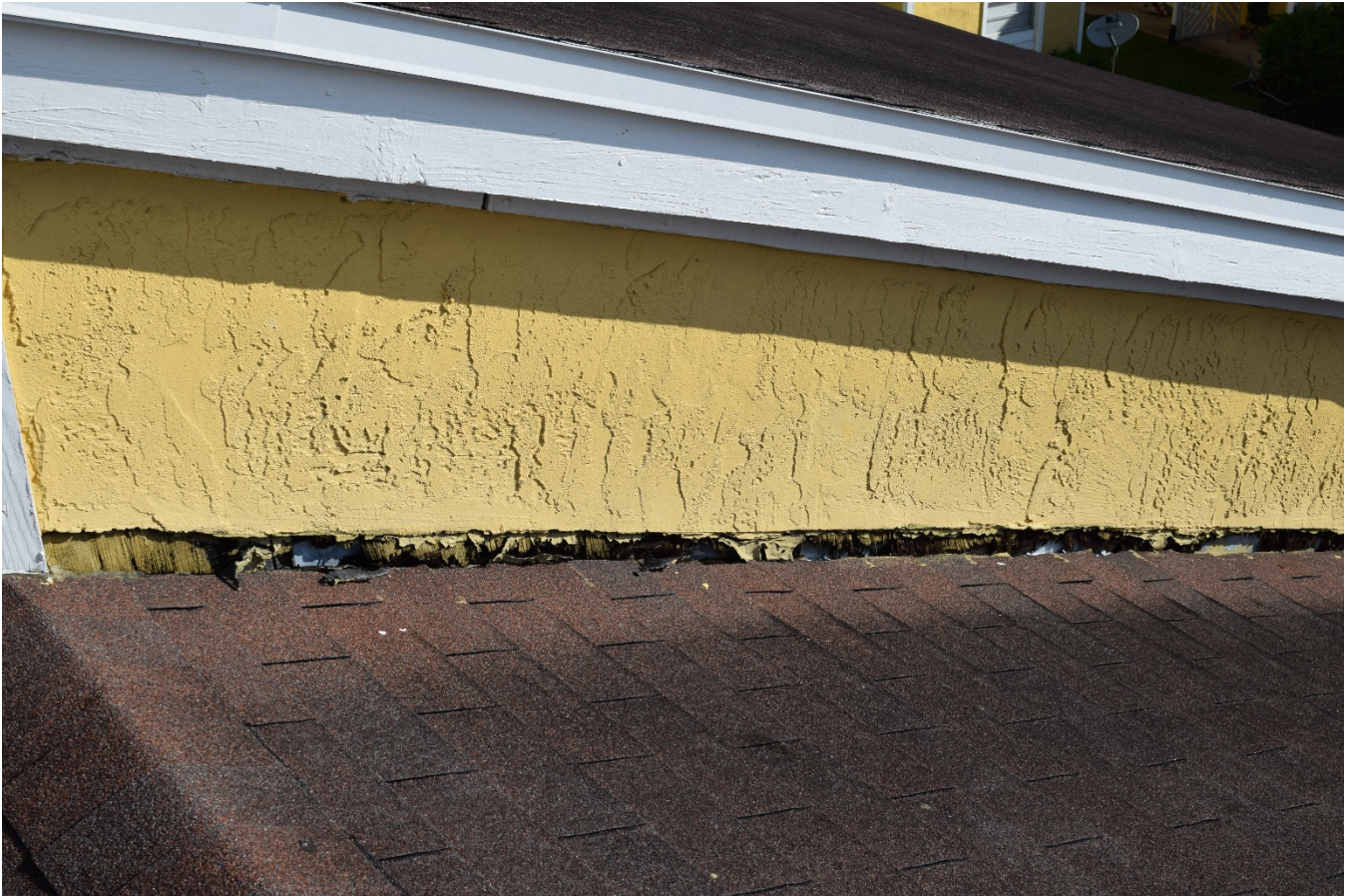
Remove stucco to install new weep and step flashing
