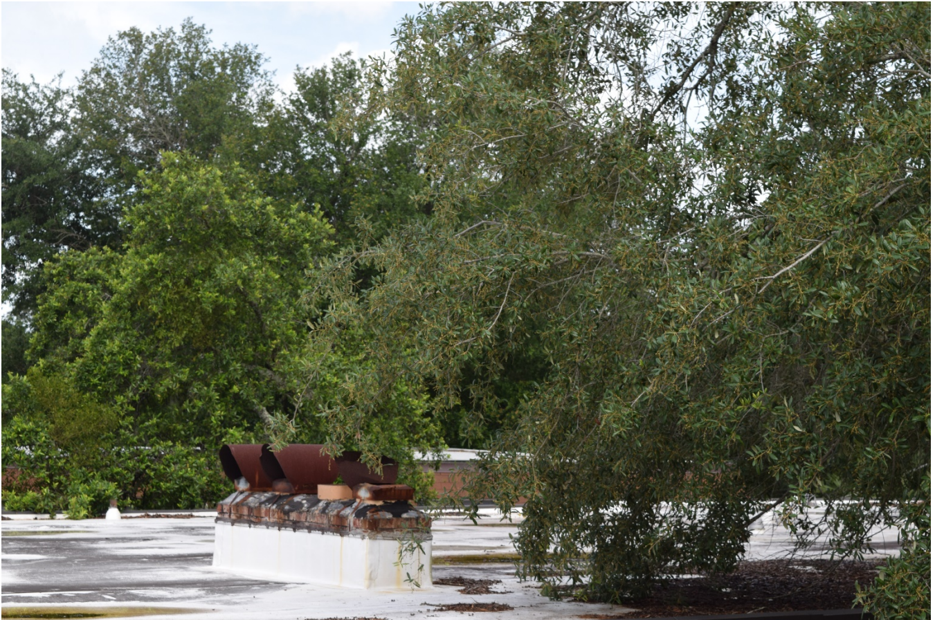
Install new or fabricate sheet metal tops for roof vents
