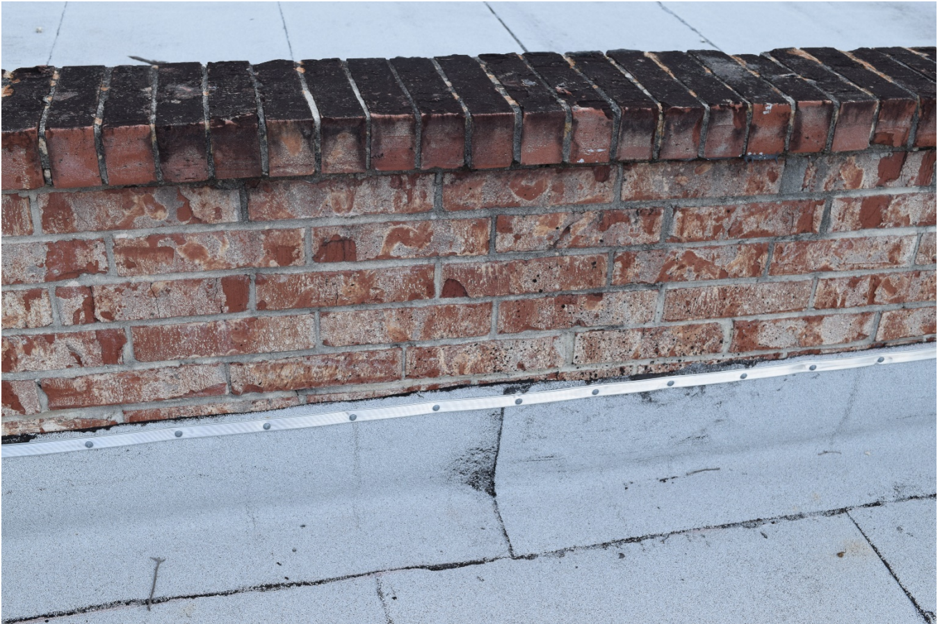
Clean Term-Bar and seal term-bar to brick per NRCA guidelines
