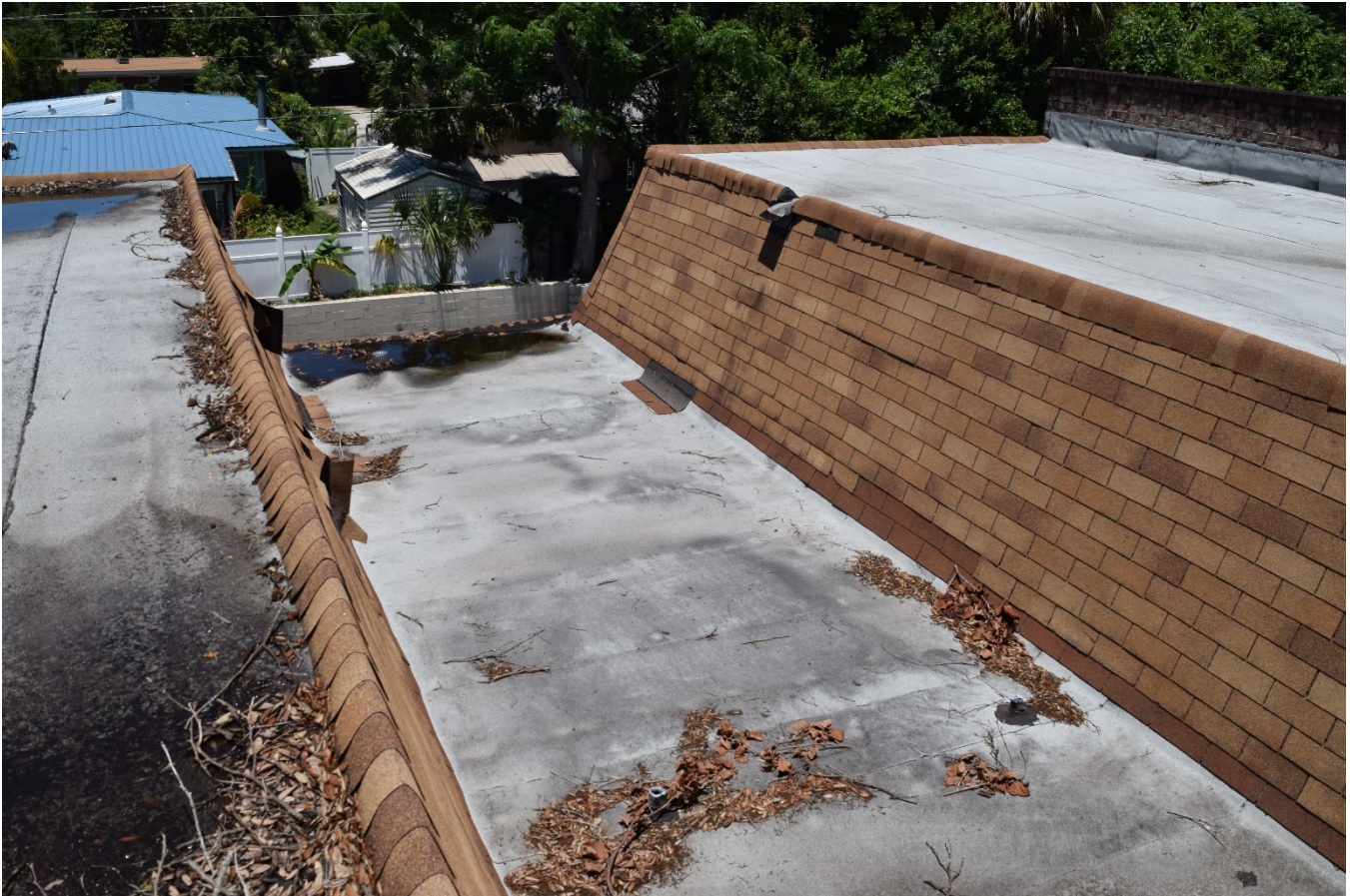
Clean debris from low slope roofs and around drains
