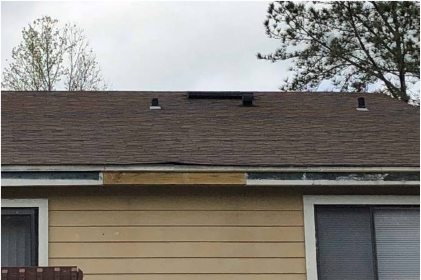
Prep, prime and paint existing unpainted fascia
