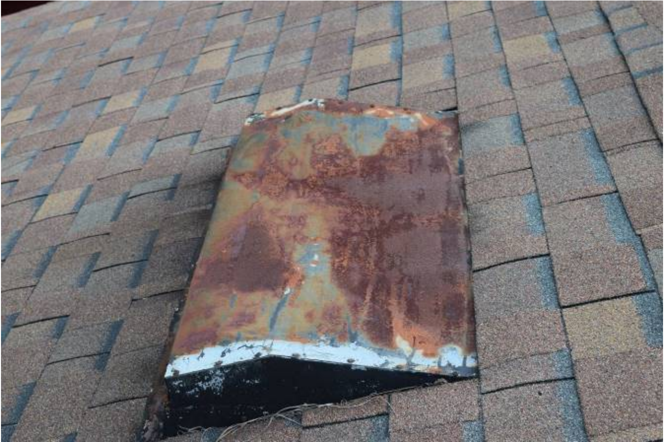
Remove and Replace dormer vents
