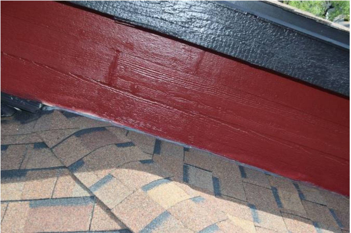
Remove siding to install new step-flashing and raise 1-1/2 to 2 inches above roof
