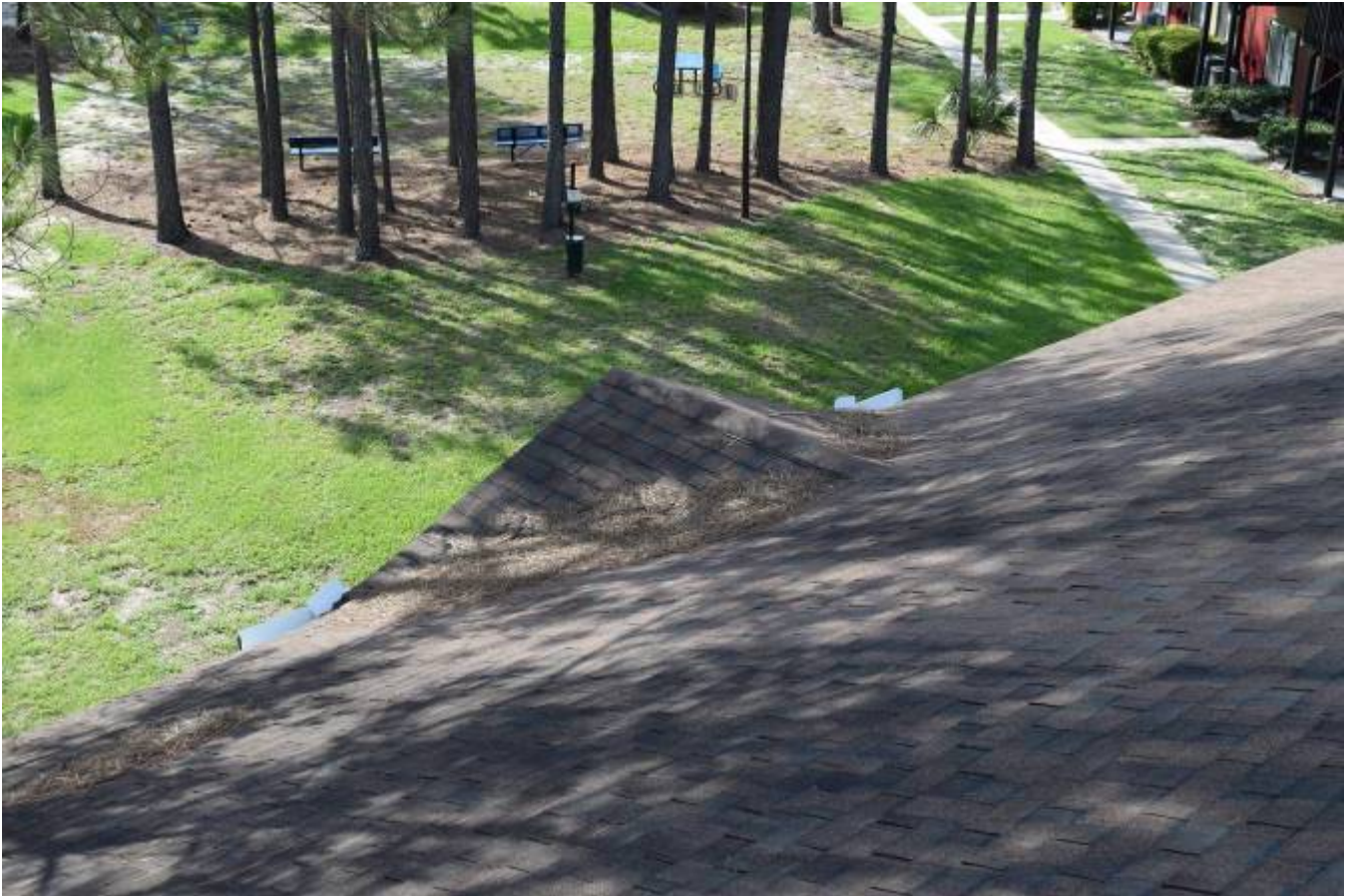
Install metal open valley
