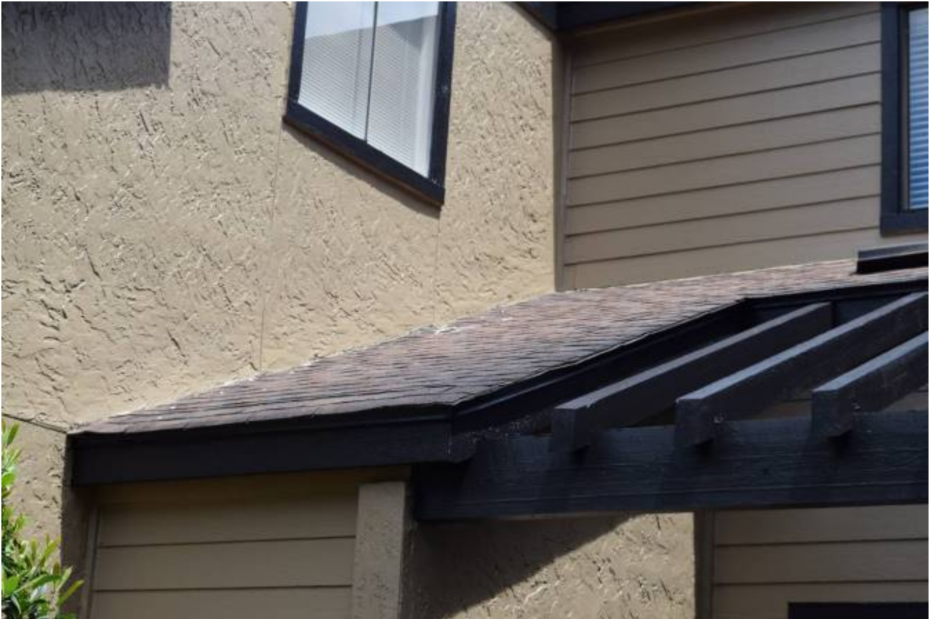
Cut stucco and install new stucco weep and step-flashing
